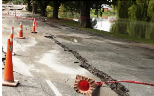
Figure 2. Lateral spreading beside lowland rivers.
