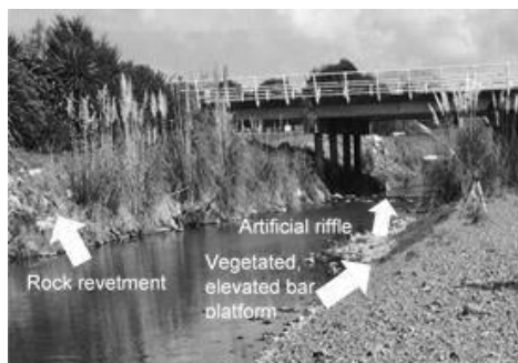
Figure 1. Annotated photograph of key morphological influences at the gravel bar studied in the Whakatiwai River.
